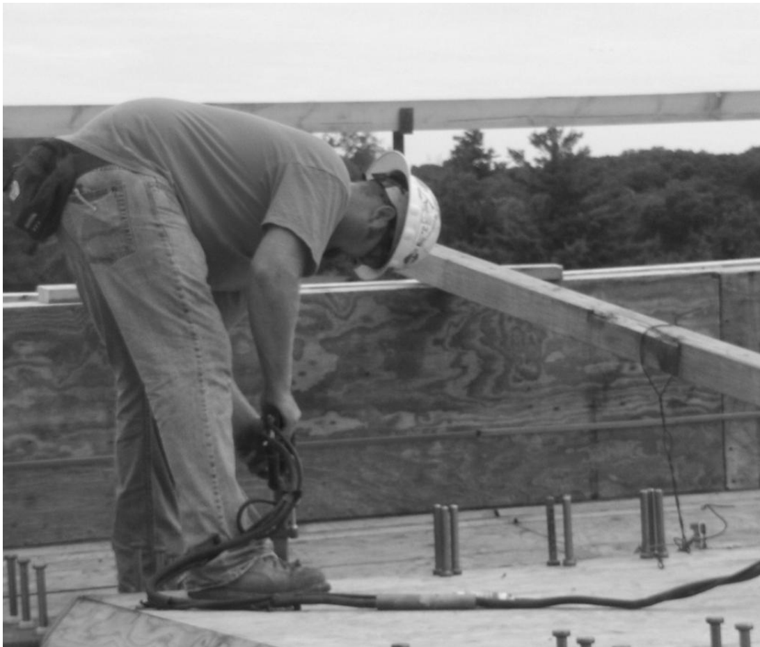
Figure 38. Posture maintained during traditional stud welding
